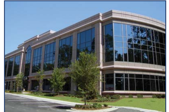
Halcyon Point Buildings B and C
