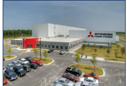
Mitsubishi Power Systems Turbine Manufacturing Plant
