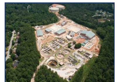
Yellow River Water Reclamation Facility
