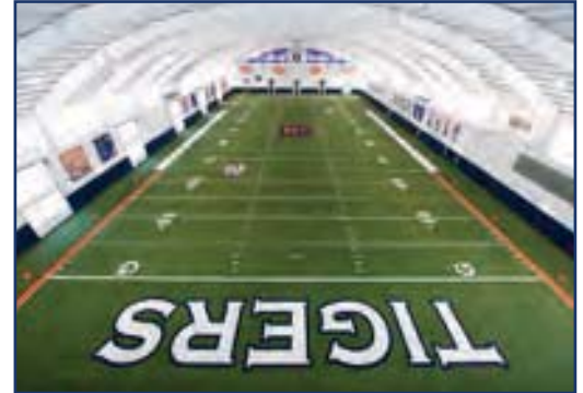
Auburn University Indoor Football Practice Facility
